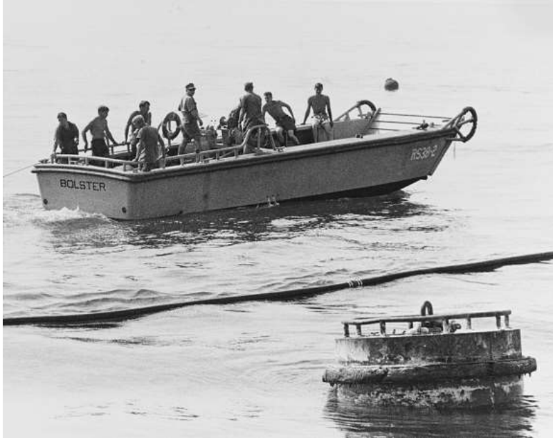
Bolster's dive boat towing a repaired four-inch fuel line into position. The line will rest on the sea floor for tanker transfer of fuel ashore. Off the coast of Vietnam, July 1965. National Archives photograph #USN 1139765
