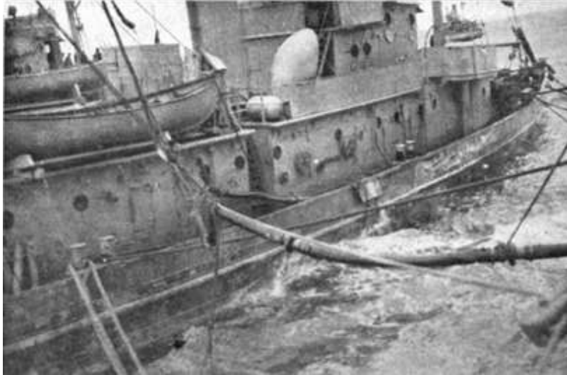
USS Pelican being kept afloat by a pumping hose from sister ship USS Eider . The Northern Barrage (Taking Up the Mines) (Washington, DC, 1920)
