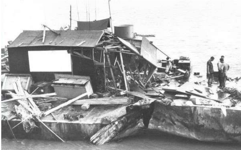
Pontoon and guard shack wrecked by two exploding mines attached to Westchester County's hull evidence the force that opened her hull, killing and wounding many sailors and soldiers sleeping in adjacent berthing spaces. Courtesy of Albert Moore
